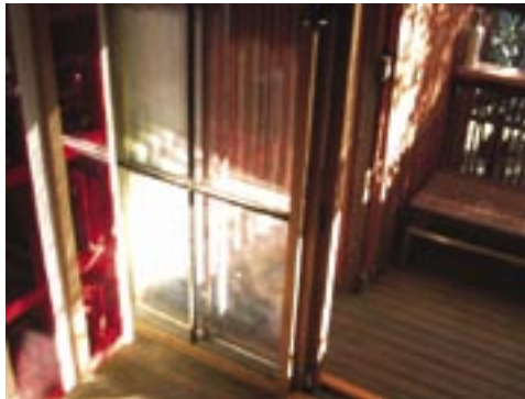
Figure 7: Edges, materials, protrusions, 2004. (Photography: Matthew Dixon)
