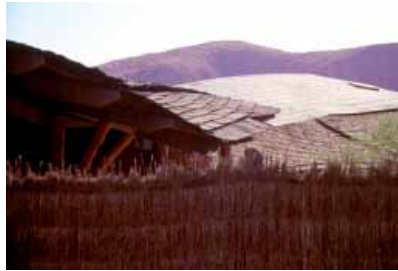
Figure 1: Exterior of cultural centre. (Photography: Jillian Walliss)
